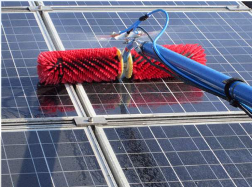
Fig. 8. Washing of the PV installation
