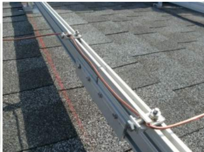
Fig. 7. Fragment of the lightning installation in the PV system
