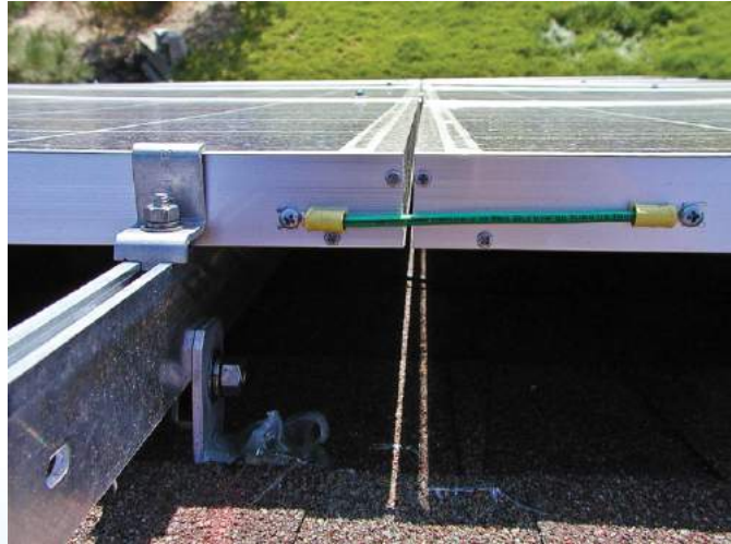
Fig. 7. Connection equalising potentials of module earthing in PV systems
