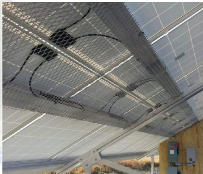
Fig. 6. Proper connection of the PV cables with use of plug connectors
