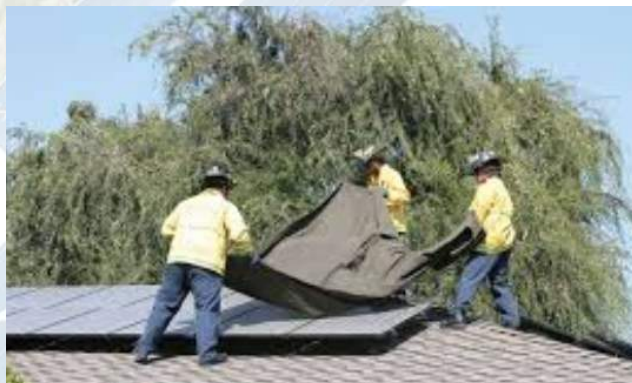
Fig. 4. Protection of the PV module with the tilt
