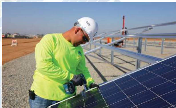
Fig. 1. Installation of the mechanical structure for the ground-based PV system
