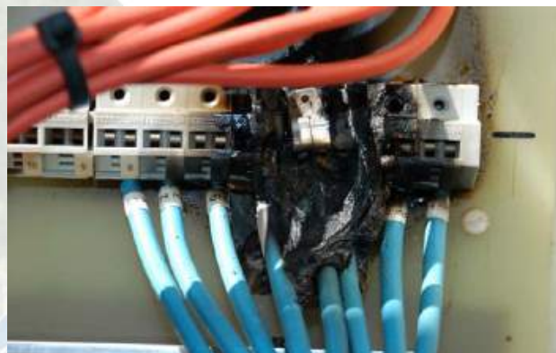
Fig. 8. AC switchboard fire in the PV installation
