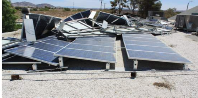
Fig. 3. Damage of the PV generator under the influence of wind
