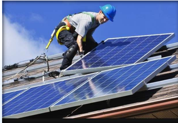
Fig. 2. PV system fitter working at a height at the module installation
