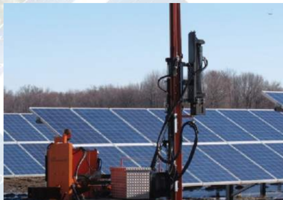
Fig. 1. Pile driver to drive ground structures
