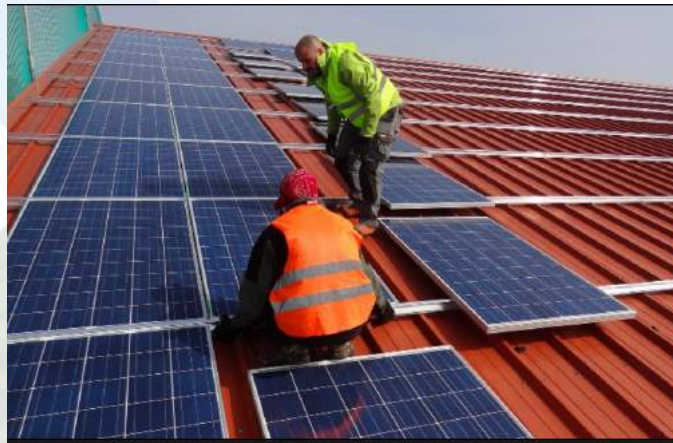
Fig. 5. Assembly of modules on the roof supporting structure
