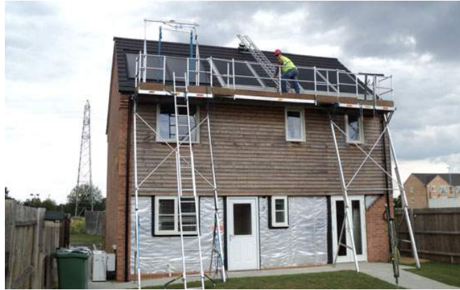
Fig. 3. PV system fitter working at a height
