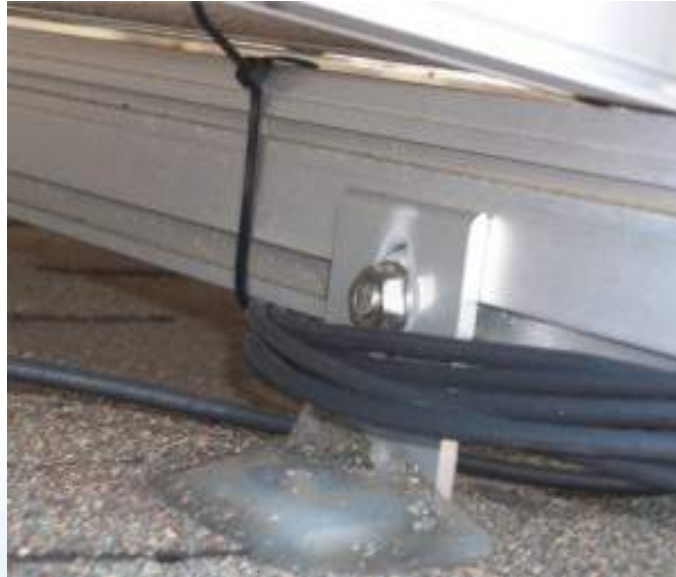
Fig. 5. Incorrectly arranged PV cables without the cable route
