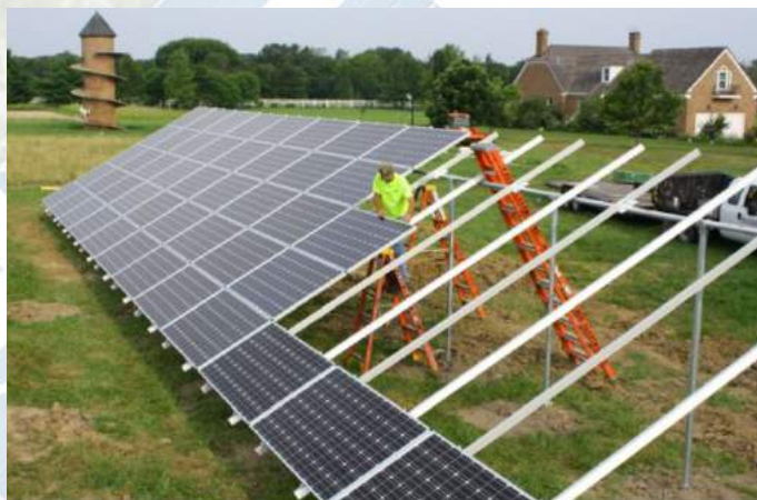
Fig. 6. Assembly of modules on the ground supporting structure
